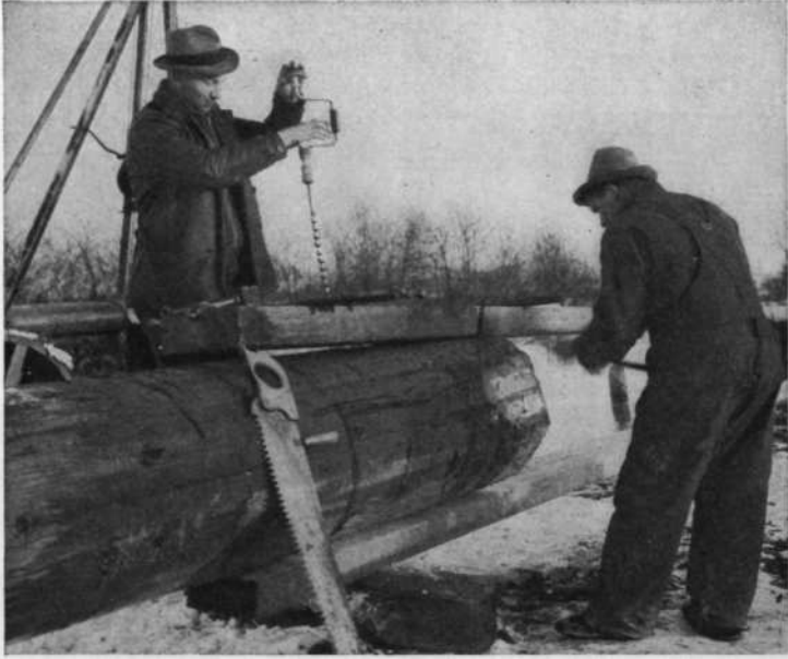
FIG. 3.112. The beginning of a pole-splicing operation and the construction of a butt-spliced pole. (Photograph courtesy of National Broadcasting Company.)
