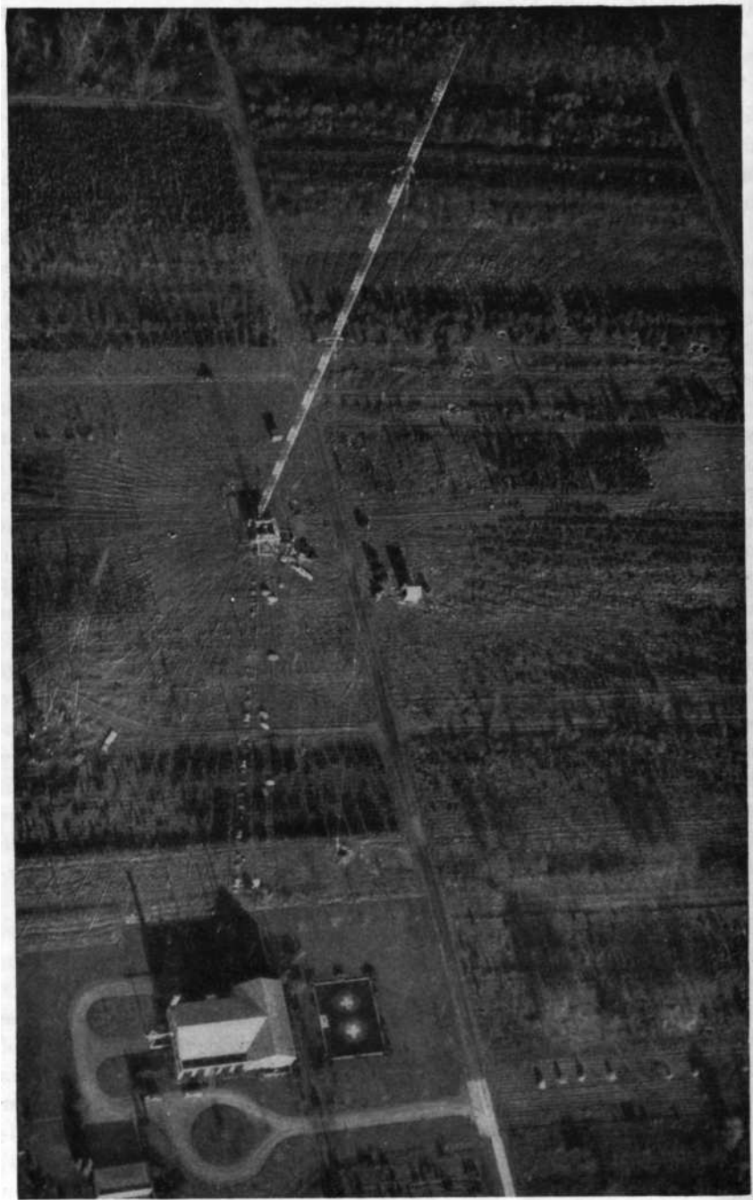
FIG. 2.52. Aerial view of a high-power broadcasting station (Radio Station WJZ when it was located at Bound Brook, New Jersey), showing the station building, the 750-foot radiator, and the freshly furrowed ground where the ground wires were plowed into the soil. (Photograph courtesy of National Broadcasting Company.)
