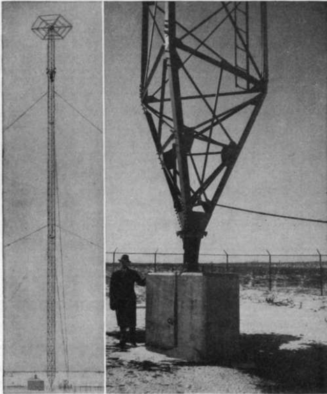
FIG. 2.55. A top-loaded sectionalized guyed vertical radiator and its base detail. Radio Station WMAQ, Chicago, Illinois. (Photograph courtesy of National Broadcasting Company.)
