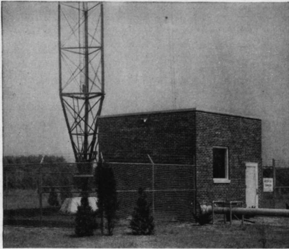
FIG. 2.54. Base of a guyed broadcast vertical radiator, coupling house, protective fence, and the 10-inch concentric transmission line suitable for 500-kilowatt service. Radio Station WJZ at Bound Brook, New Jersey (location now at Lodi, New Jersey). (Photograph courtesy of National Broadcasting Company.)
