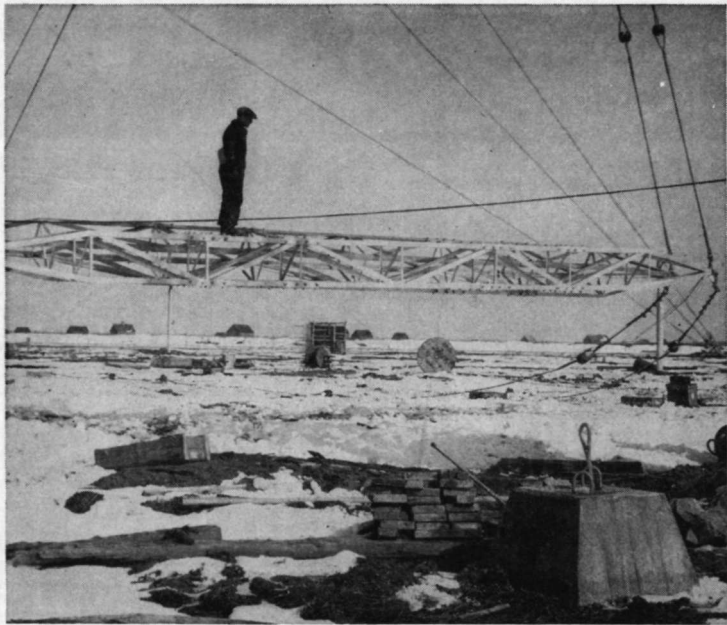
FIG. 3.101. Fabricated spreader used to space the radiator and reflector curtains of a large dipole array in the main catenary, shown before being raised into the air. This is part of the array used for 6-megacycle broadcasting. (Photograph courtesy of Canadian Broadcasting Corporation.)
